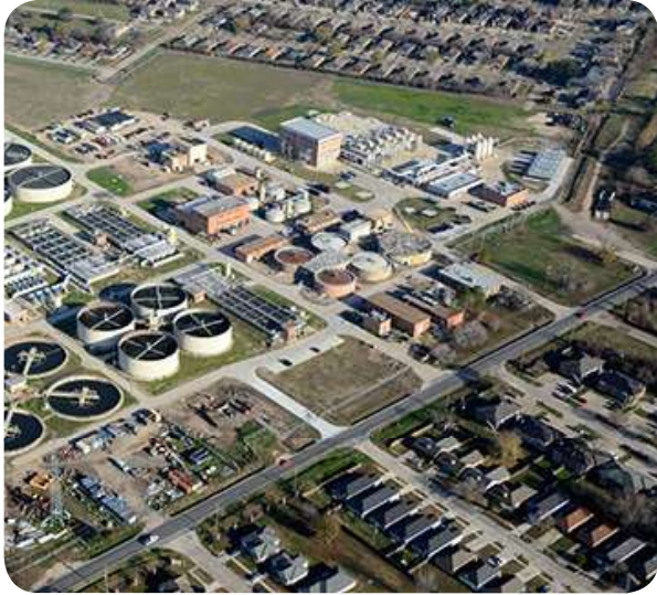
South Wastewater Treatment Facility
